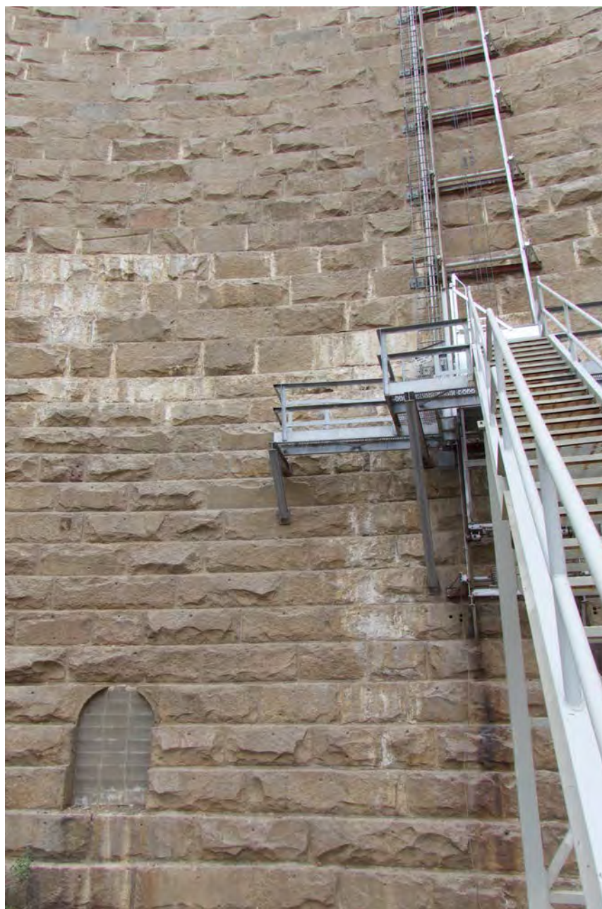
Photo #46: Stonework detail and plugged access gallery, downstream face Pathfinder Dam. Camera facing west.
