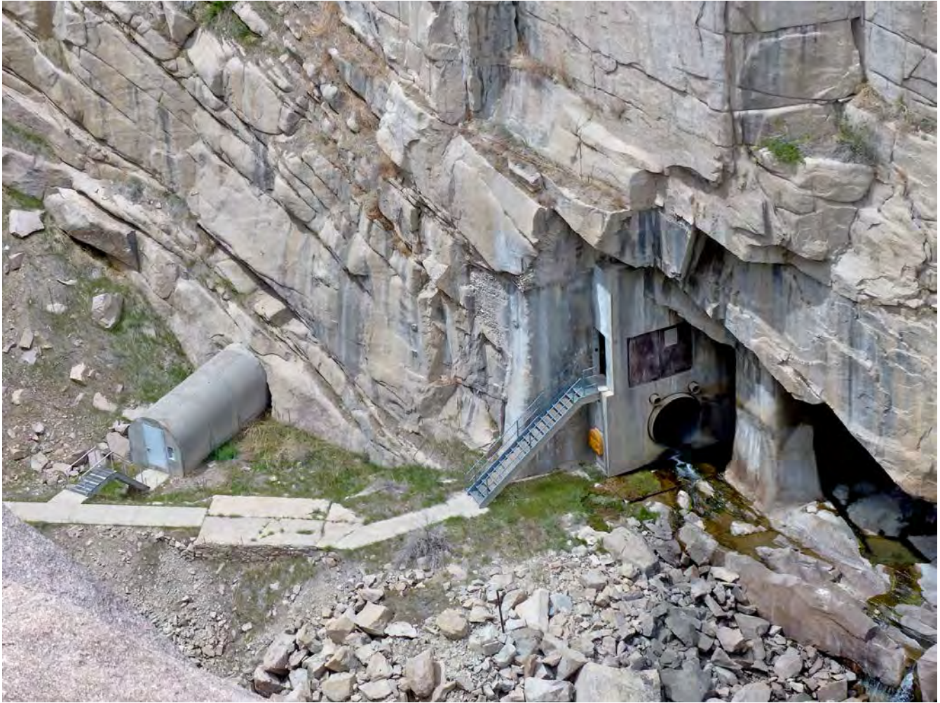
Photo #10: Canyon floor below Pathfinder Dam, north side of river, showing the access structures to the high-pressure gates (Quonset hut to left) and the river outlet works control house (right in canyon wall), and the outlet for the 60-inch Jet-Flow valve (all part of Feature E, non-contributing). Camera facing downward and northwest.
