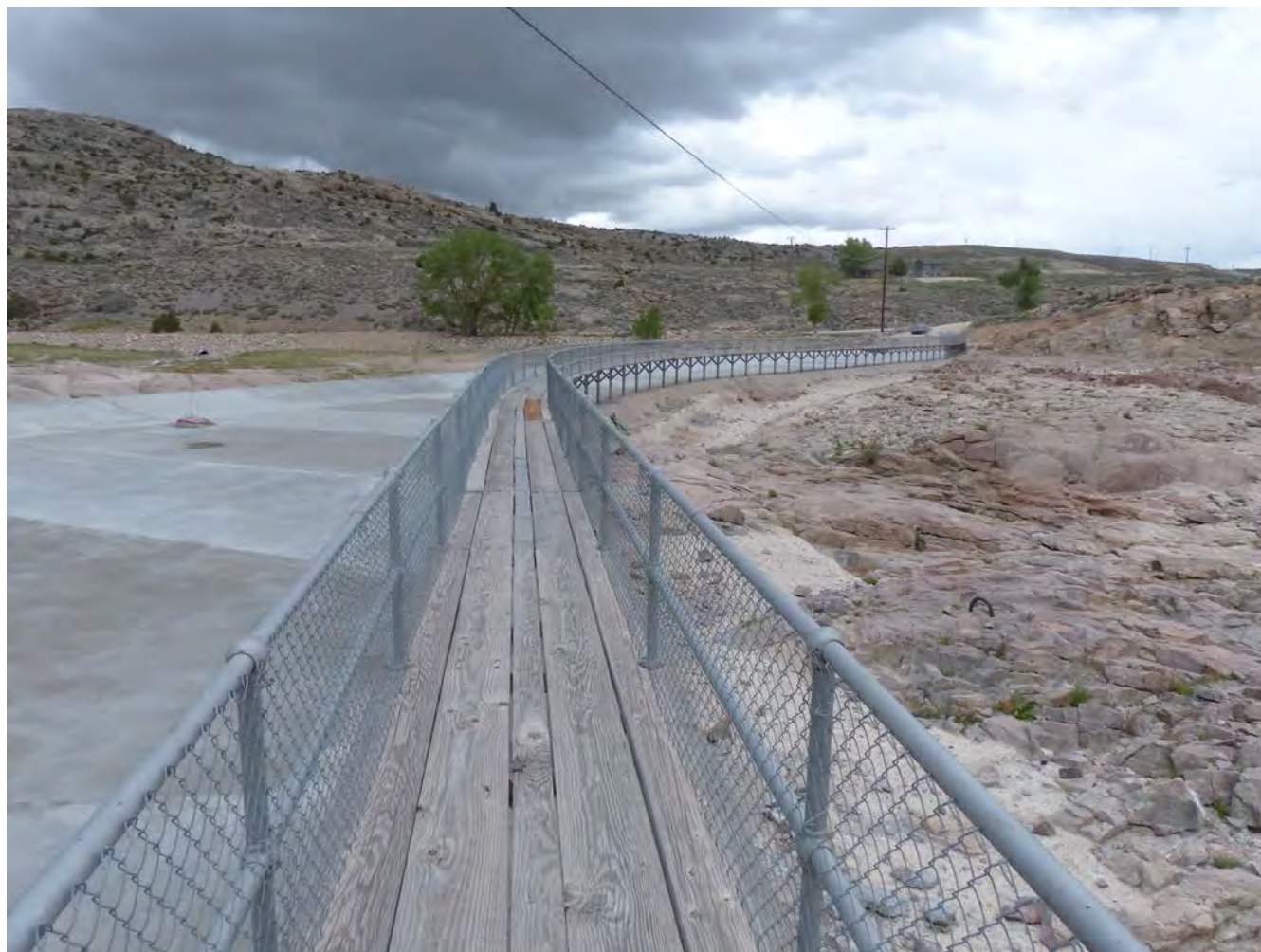
Photo #32: New spillway concrete ogee weir and apron (left, Feature J, non-contributing), facility access walkway (center, Feature I, non-contributing), and upper end of natural section of Pathfinder spillway (right, Feature H, contributing). Note the U-bolt set into the spillway bedrock. Camera facing north.
