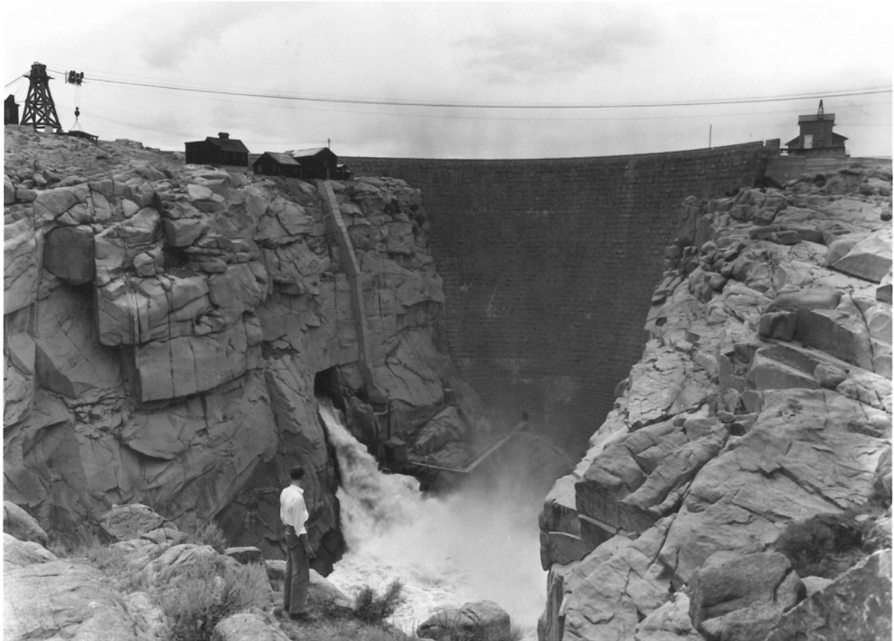
Historic Photo #22: Pathfinder Dam, 1940, view looking west at the dam's downstream face. Note the 1920 cableway (extant today), walkway from dam gallery to south outlet tunnel valve house (no longer extant) and south access ladderway (largely extant), and buildings (no longer extant) at the south abutment. Also note Sluice Gatehouse (upper right, extant) still have the gate operating superstructure that was removed during the 1990s north tunnel outlet works renovations.
