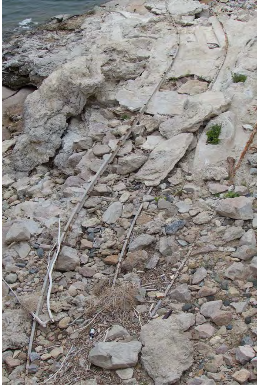
Photo #50: Last known remnants of rail system (Feature R, contributing structure) used to haul blocks from the quarries to the dam. It is located next to the dam's upstream face just below the Emergency Gatehouse. Camera facing down and to the west.
